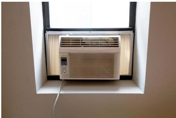
Window units have all of the components housed in one box. Window units tend to be noisy because the compressor (*which is a part of the condenser*) is noisy.
