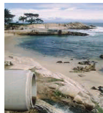
A storm drain leading to the coast.
