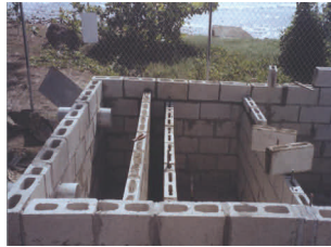
Holding tanks under construction
