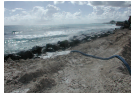
Site water being discharged to the sea
