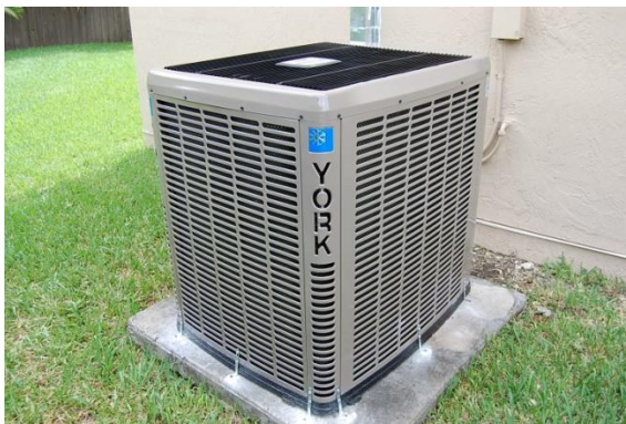
Figure 2: Condensing component of an air-handling unit. This is usually located on the roof of a building
