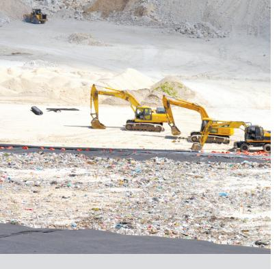
which utilizes a liner to prevent buried waste and leachate from coming in contact with underlying soil and groundwater. This reduces the risk of environmental contamination due to improper disposal of the waste.
