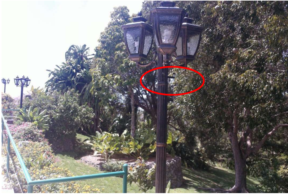
Figure 7: SO 2 /NO 2 and Ozone Samplers on light pole at Gun Hill Signal Station
