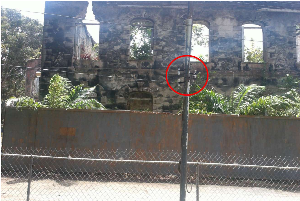
Figure 5: Tubes placed on disused flagpole adjacent to the Great House ruins at Farley Hill National Park
